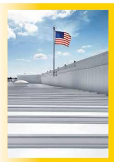
Roofs have it hard. On an 89° day, a typical black roof can experience a 100° variation from 175° at the hottest peak to 75° ambient temperature at night. This constant temperature fluctuation and UV exposure can create tremendous strain over time. Most commonly, roofs fail where dissimilar materials meet at penetrations, seams and edges. Minor structural issues can cause additional challenges such as poor drainage and ponding water.
